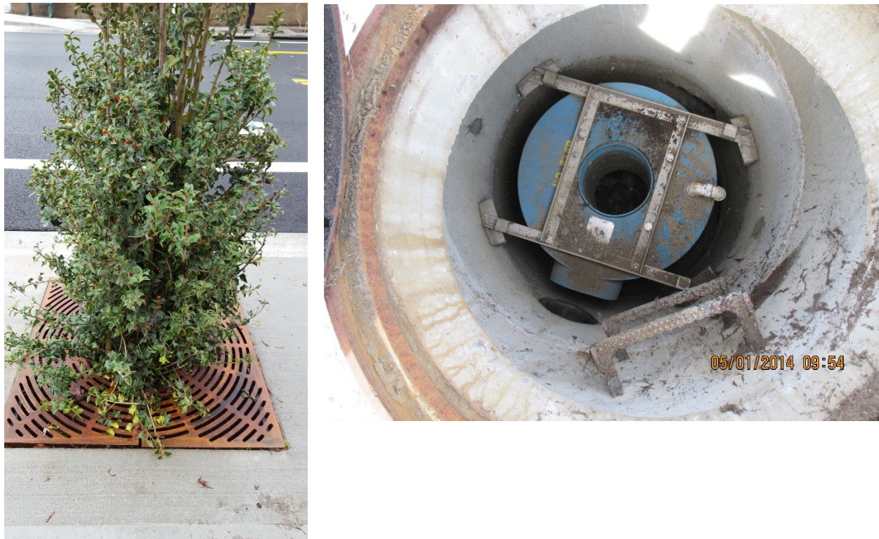
Figure 4.11. Filterterra Units (left) and Filter Cartridge Units (right) are examples of proprietary Treatment devices that meet the requirements of this Design Manual.
