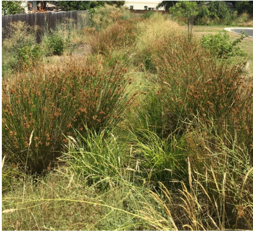
Figure 4.6. A Water Quality Swale with dense mature vegetation that provides filtering of stormwater runoff.
