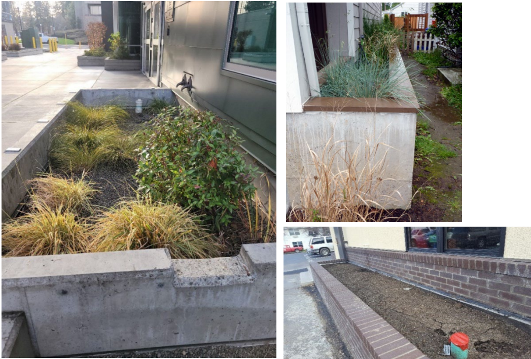
Figure 4.5. Stormwater Planters located flush with a public building (left), a fully-lined residential above-ground Stormwater Planter with an underdrain (upper right), and a newly constructed above-ground Stormwater Planter with an underdrain (lower right).
