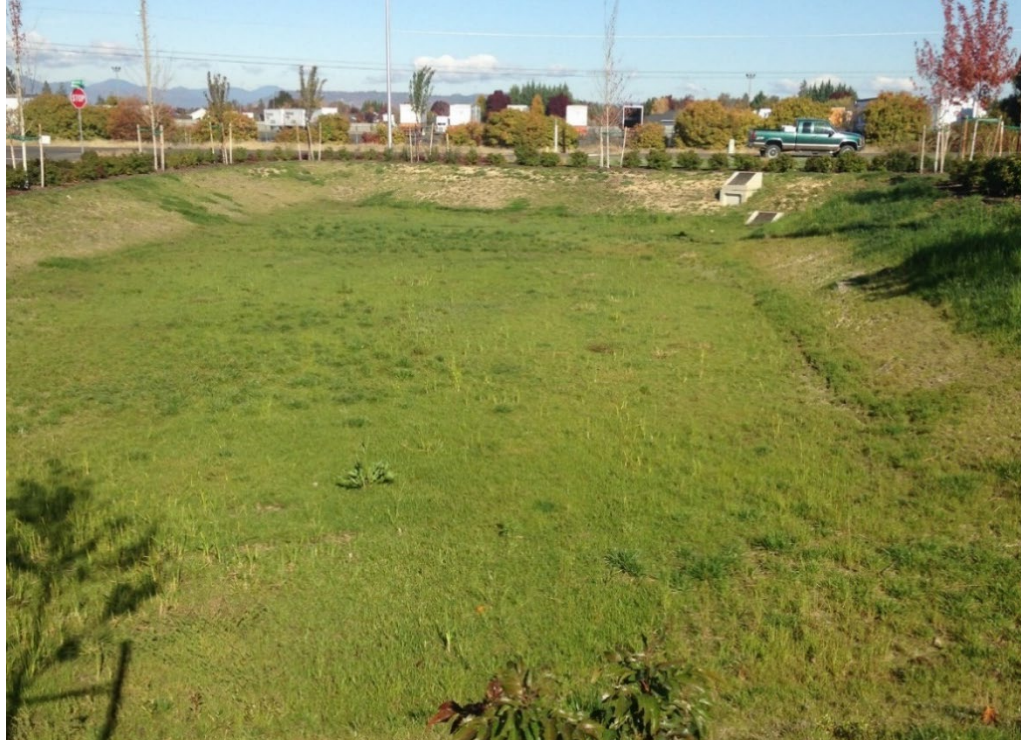
Figure 4.13. A Detention Basin designed to capture and temporarily hold Peak Runoff that is then slowly released through the control structure.
