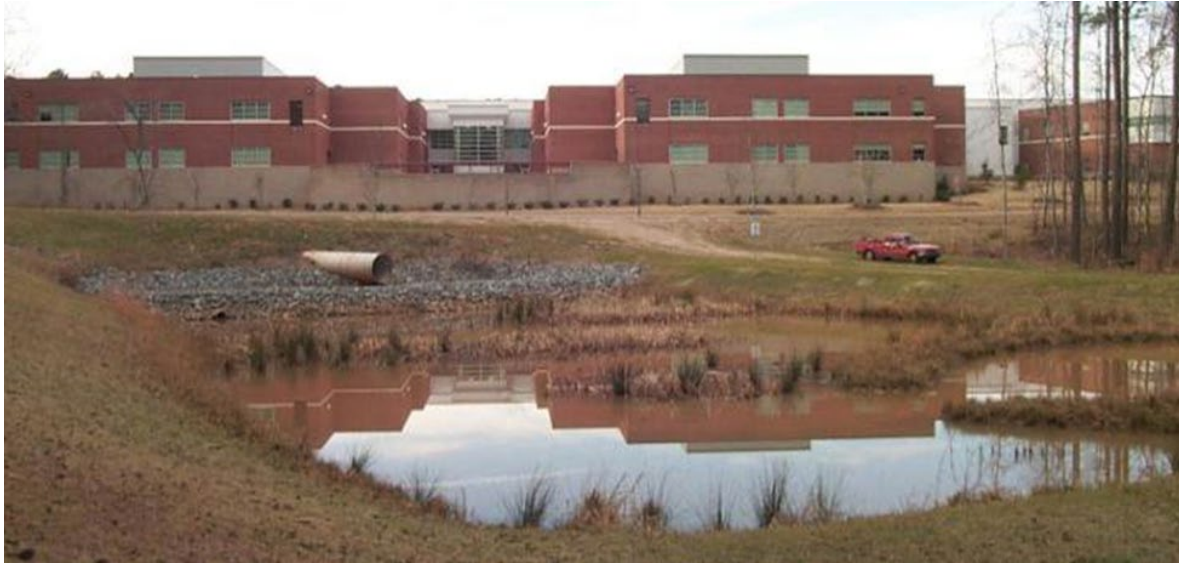
Figure 4.10. Example of a Water Quality Settling Basin with a vegetated baffle system to lengthen the distance from the inlet and outlet.
