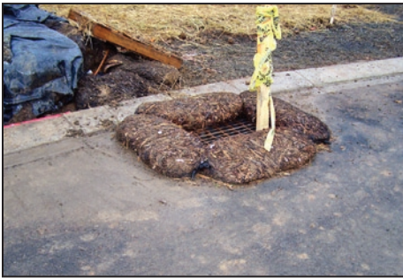
Source: Clean Water Services
