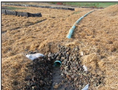
Source: Clean Water Services
